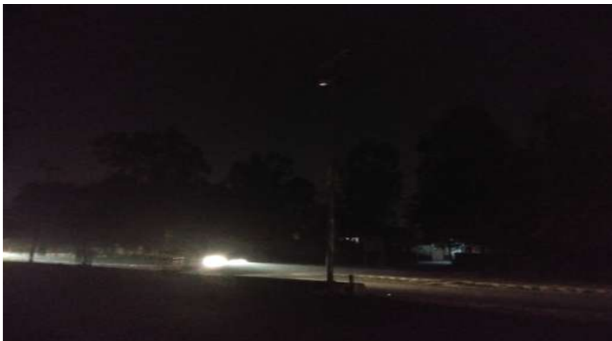
Inadequate lighting and security on the main road – Sonepat road
